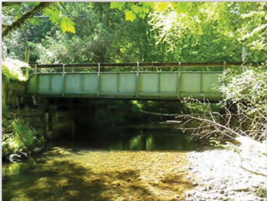
This bridge carries residents to the local community and many visitors to Lake Walker Recreational Area.
