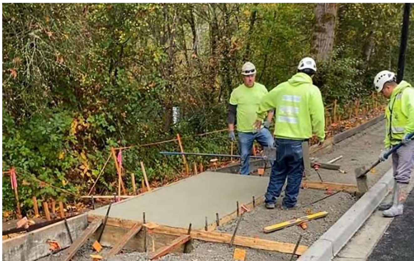
Oct. 24, 2022 – Contractor crews pour the first of many concrete sidewalk panels.
