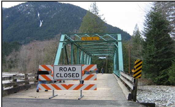
Figure 4: Bridge #999W closed for traffic- looking west
