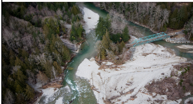
Figure 6: Aerial View of the Bridge and Washout - looking downstream- island
