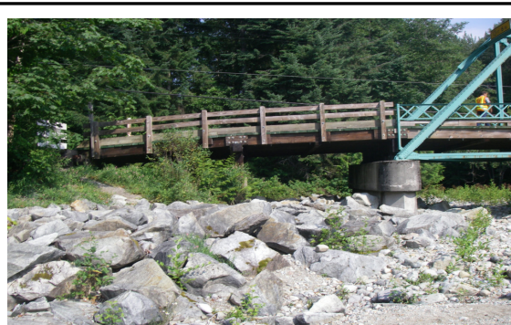
Figure 5 West Approach Spans- looking Downstream
