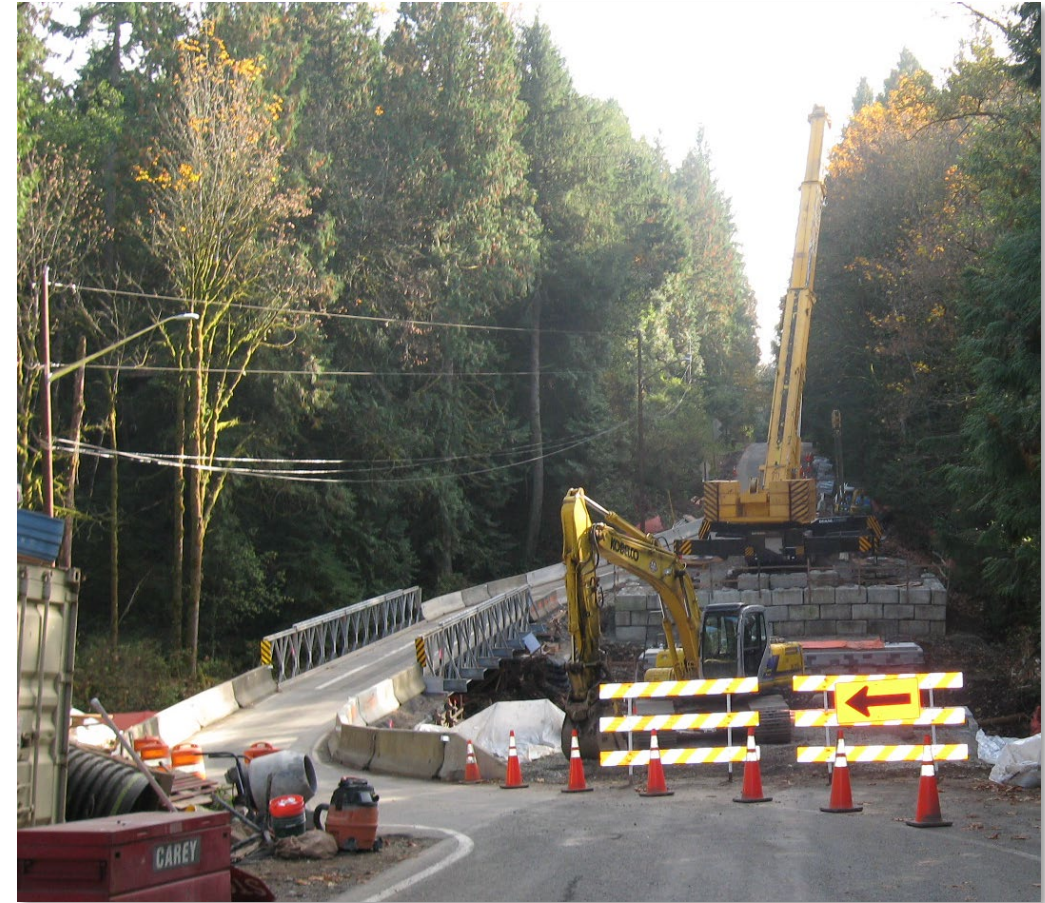
Bypass bridge from 15-mile Creek Bridge construction in 2013
