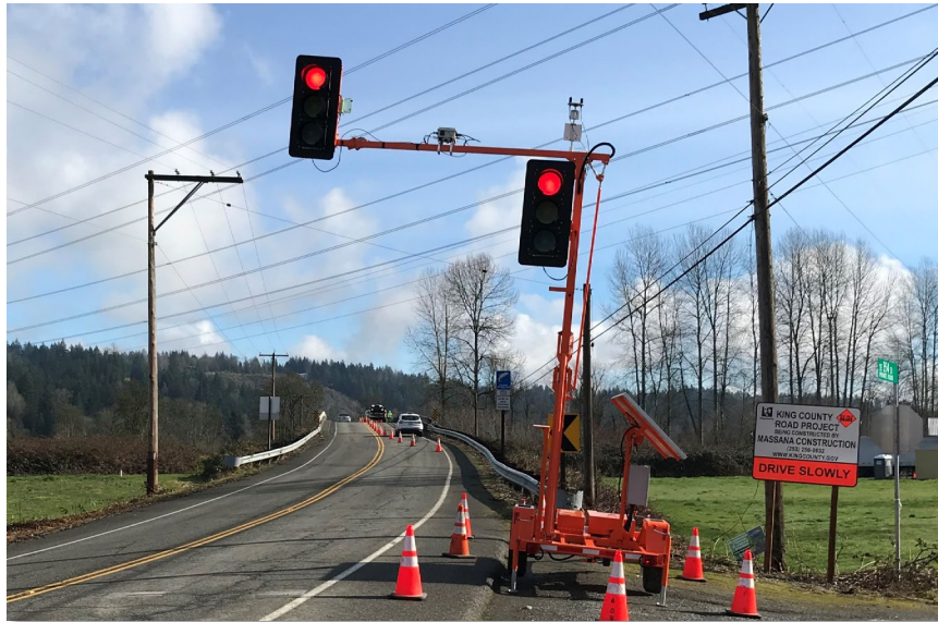
Patton Bridge Repair Project, 2021
