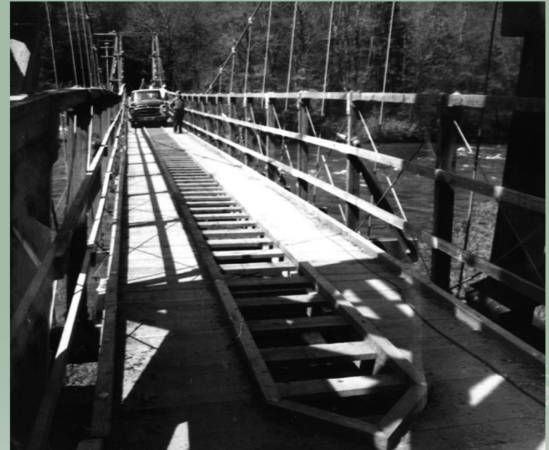
Photo of rail post-repair (1950)
