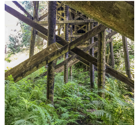
Bridge timber structure is over 100 years old.
