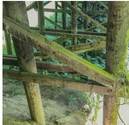
Creosote-treated timber piles are decaying.
