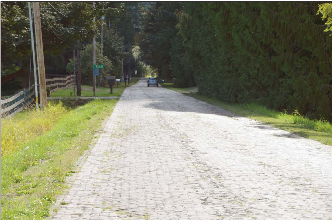
Figure 13. Parallel tracks with crushed and fragmented brick.
