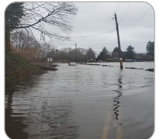
Photo caption. Southwest Quartermaster Harbor Drive, Vashon Maury Island. January 2022 storm and tidal surge over road.
