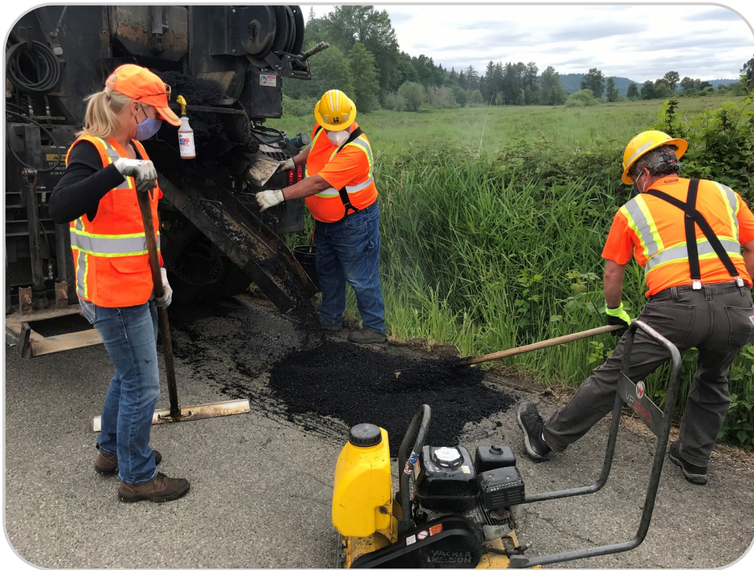
Photo caption. Road Rangers crew members delivering pothole repair services.
