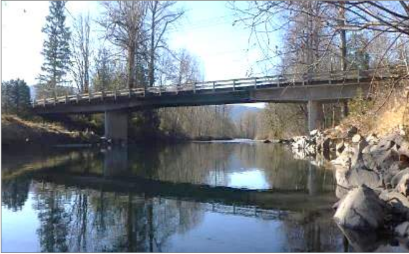
North Fork Bridge No. 122I – Looking South
