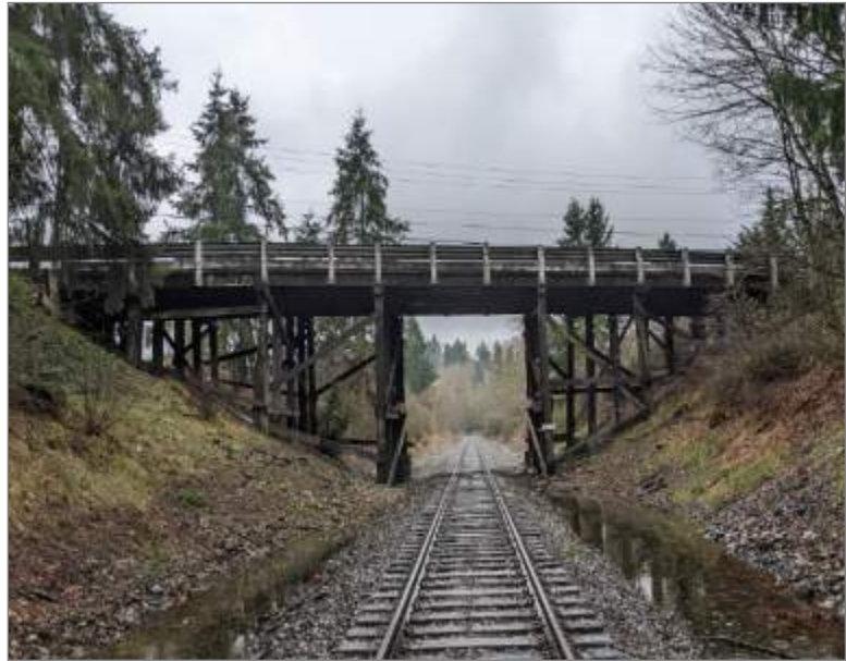
Berrydale Overcrossing No. 3086OX – Looking south near the BNSF rail-line
