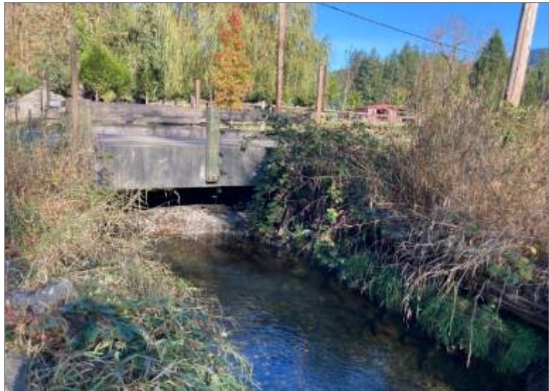
Tate Creek Bridge No. 122N – Looking North
