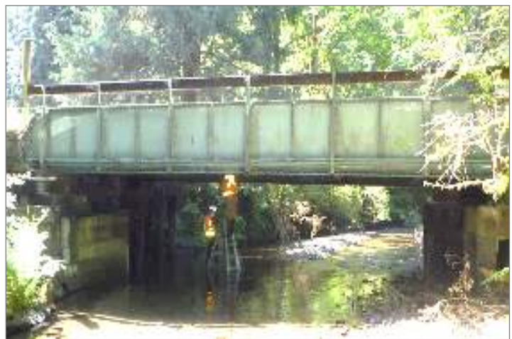
Coal Creek Bridge No. 3035A – South elevation
