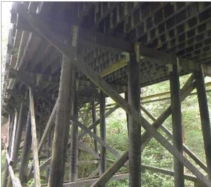
Ames Lake Trestle No. 1320A – Timber structure
