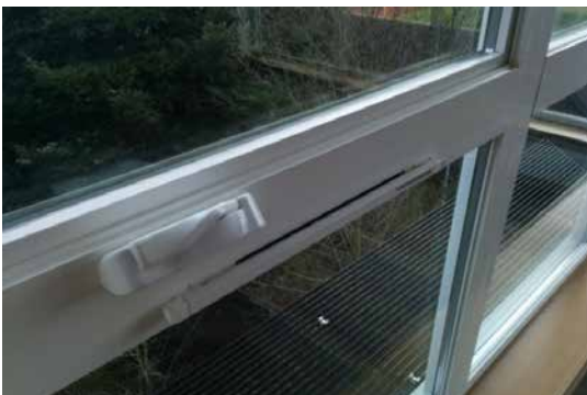
Window trickle vents are used in conjunction with whole house exhaust fans to provide fresh air ventilation. With proper planning and controls, the bathroom exhaust fan can double as the whole house exhaust fan. Source: O'Brien & Company.
