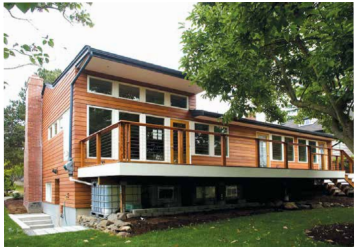
Catchment systems are available in numerous shapes and sizes, including a cube-shaped tank as pictured here. Source: Batt + Lear .
