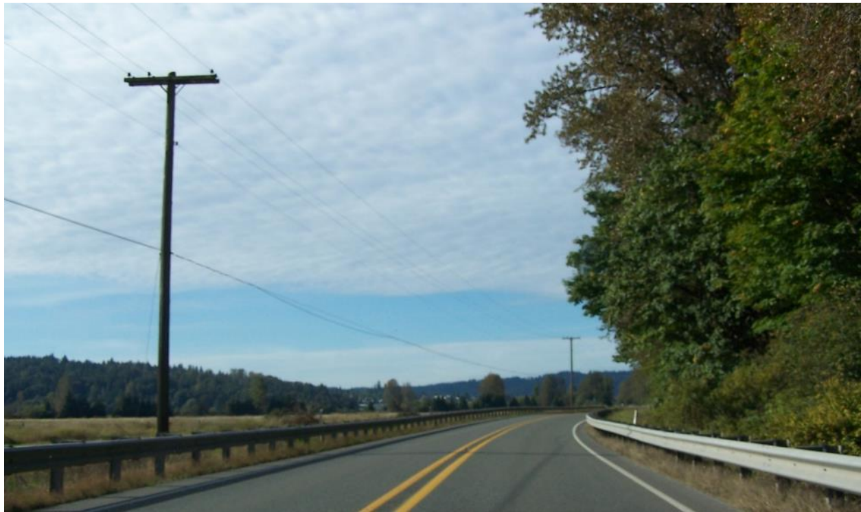
Figure 33: Typical Low-Make-Ready Pole Line in the Unserved Areas
