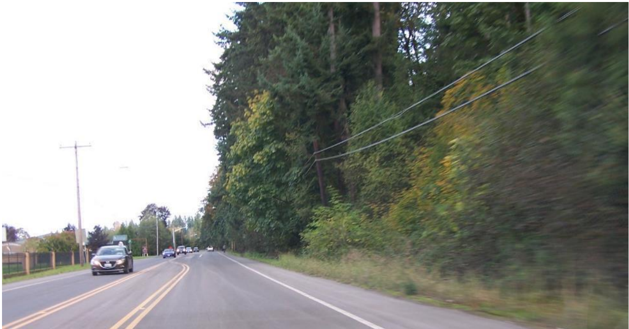
Figure 32: Pole Line Where Tree Trimming Will Be Required
