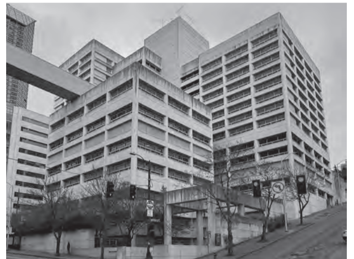
Photograph of the King County Correctional Facility, circa 2024.
