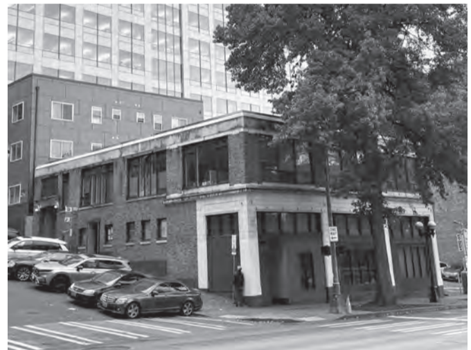
Photograph of the Yesler Building, 2024.
