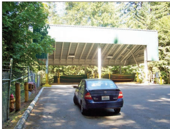
Disposal area (4 stalls) exterior gate to the Skykomish Drop Box
