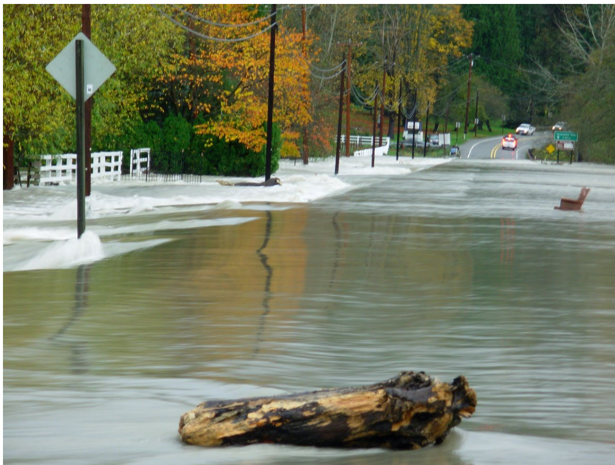
Snoqualmie River flooding of State Route 202 near Fall City, November 2006
