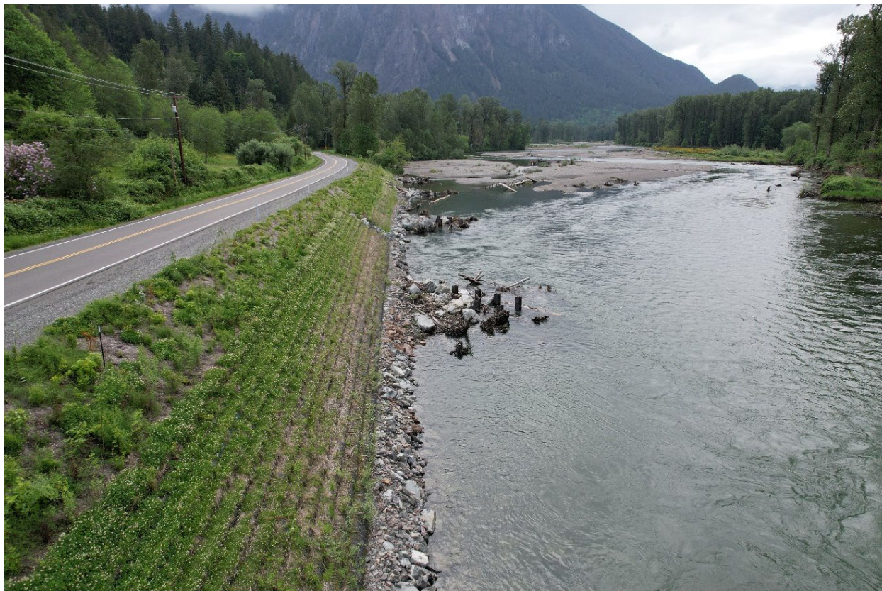
Revetment protecting Reinig Road on the Snoqualmie River, May 2023
