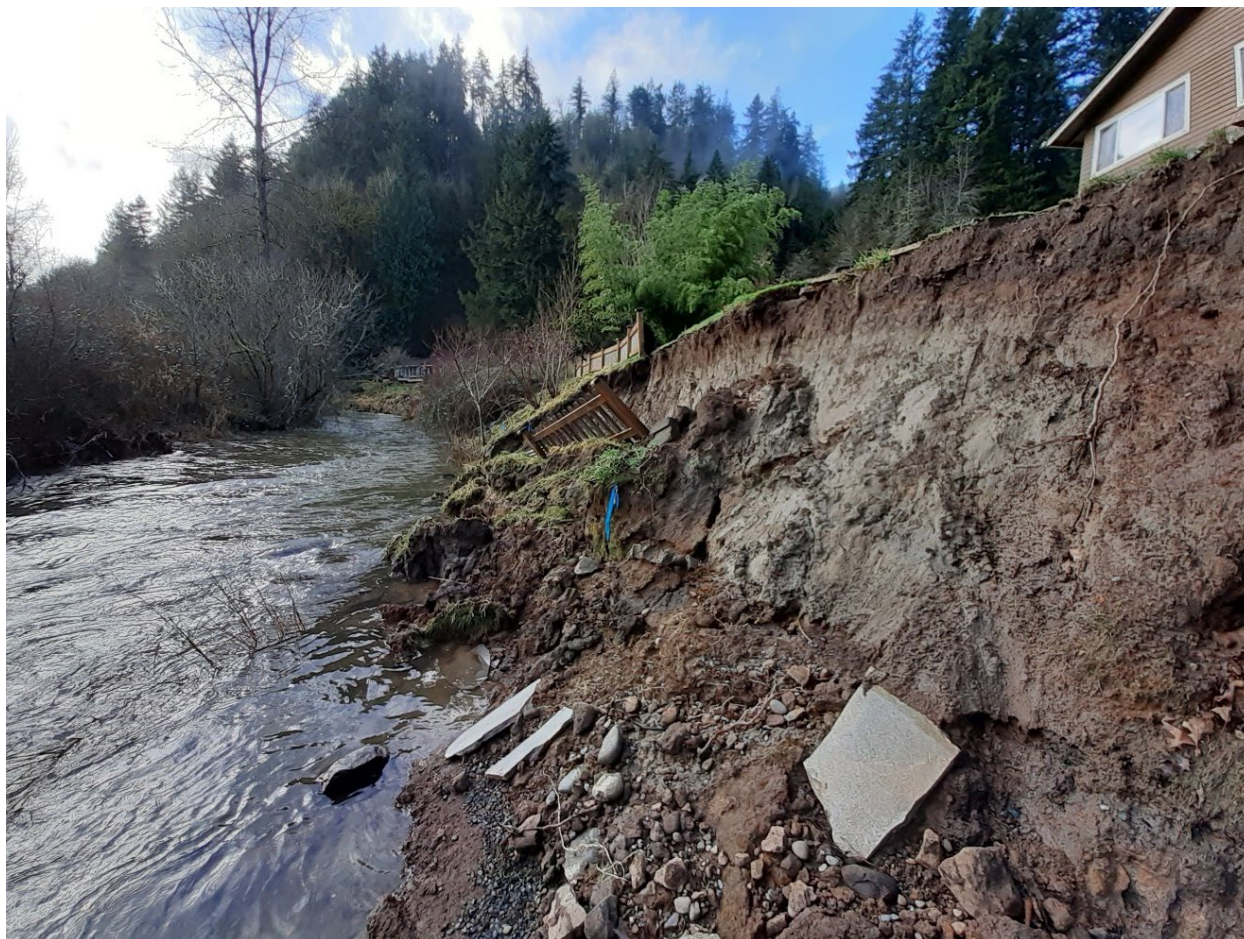
Erosion from tributary flooding on Issaquah Creek, January 2021
