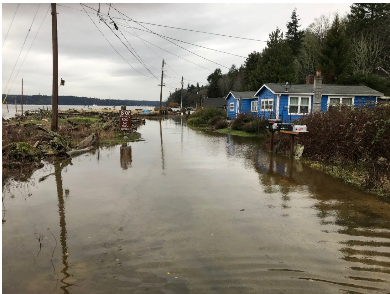
Waterfront road flooding on Maury Island, December 2022
