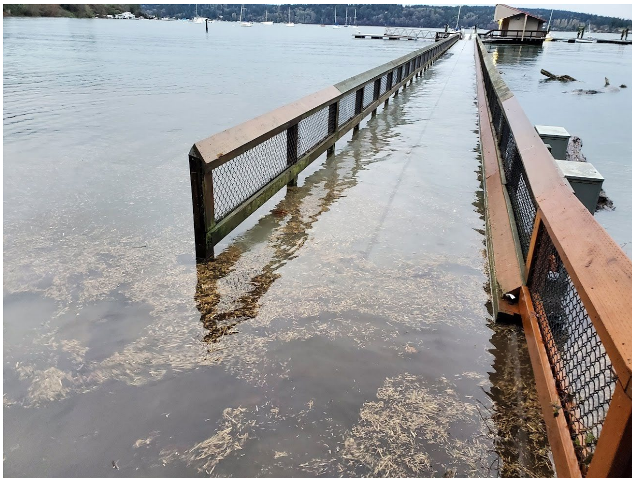
Dockton Park Marina king tide flooding on Maury Island, December 2022
