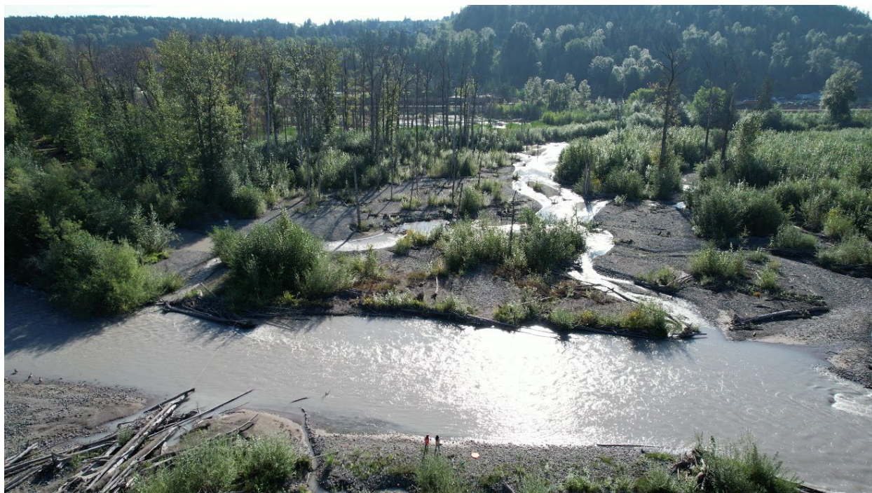
White River Countyline Floodplain Reconnection project, September 2023
