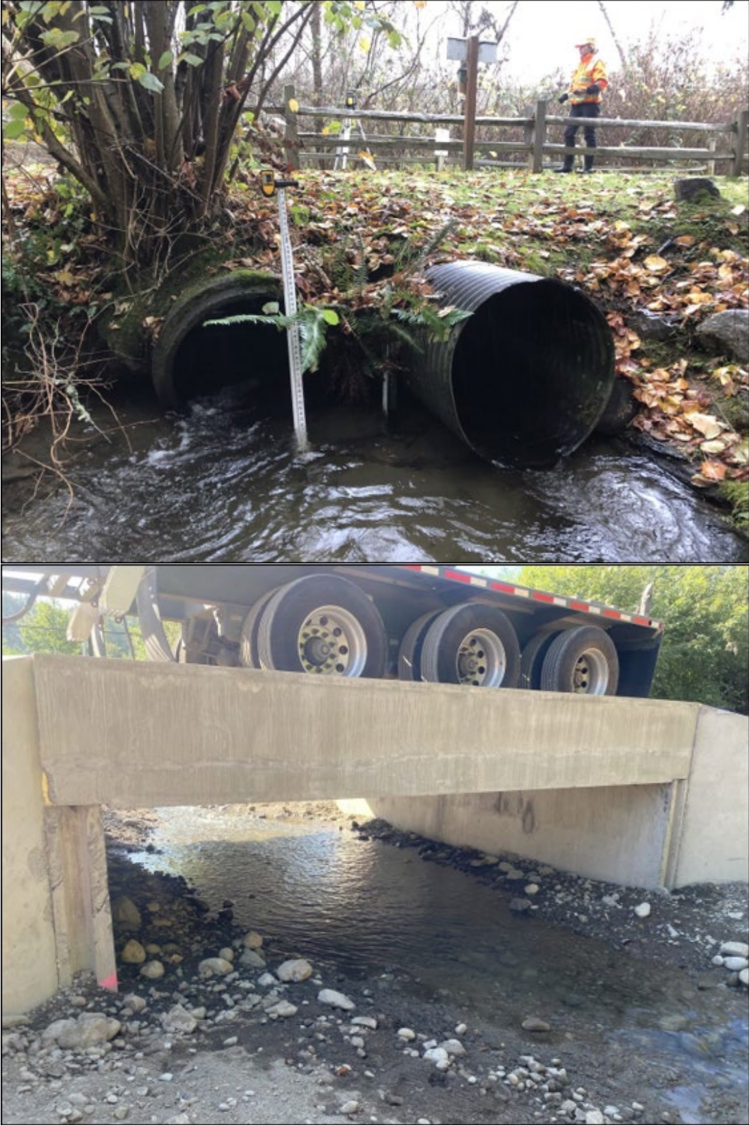
Before (top) and after (bottom): Culvert replacement with fish-friendly box culvert on Ebright Creek under East Lake Sammamish Trail, 2022
