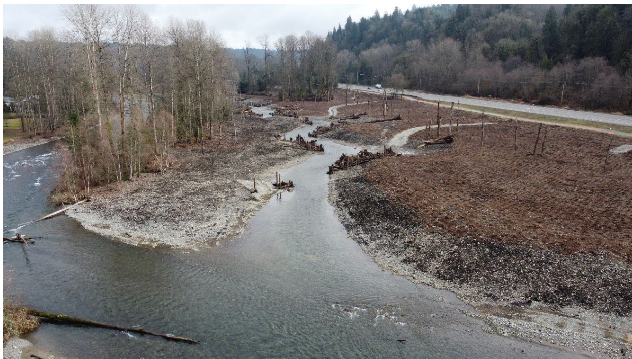
Riverbend floodplain restoration and levee setback on Cedar River, January 2023
