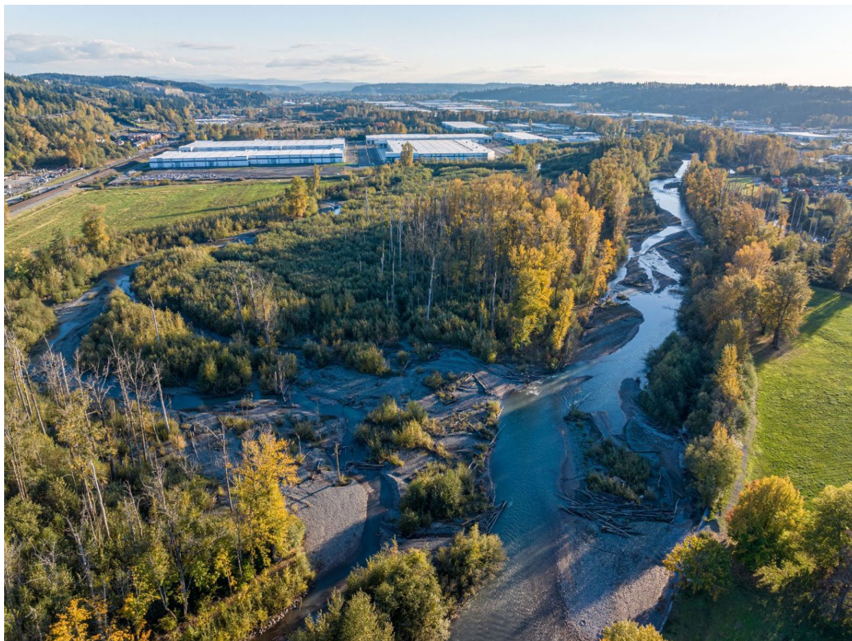
Countyline floodplain reconnection project on the White River, November 2023
