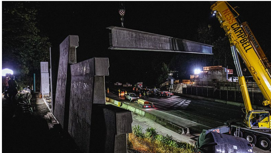
Construction of Eastrail bridge over I-405
